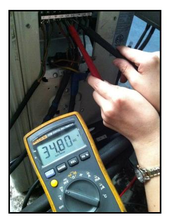
Pic 1: Use a multimeter to test the DC voltage between 2(old: L2) port and 3 port of outdoor unit. The red pin of multimeter connects with 2 (old: L2) port while the black pin is for 3 port.
